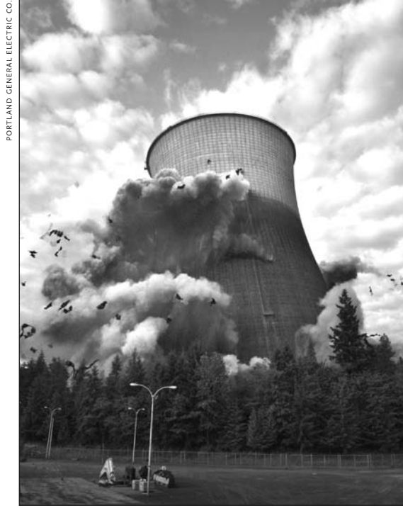
COVER PHOTO: Trojan Nuclear Power Plant demolition. Portland General Electric Company
