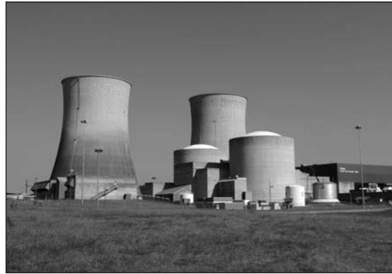
The Watts Bar-1 reactor, 60 miles southwest of Knoxville, Tennessee, took 24 years to build.
