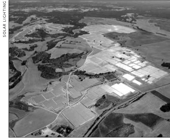
The 162,000 solar panels at Spain's 62 MW Olmedilla Solar Park (the world's largest photovoltaic power station) produce about 87.5 gigawatt-hours of electricity a year—enough to power more than 40,000 homes. The Olmedilla plant was constructed in just 15 months at a cost of $350 million.
